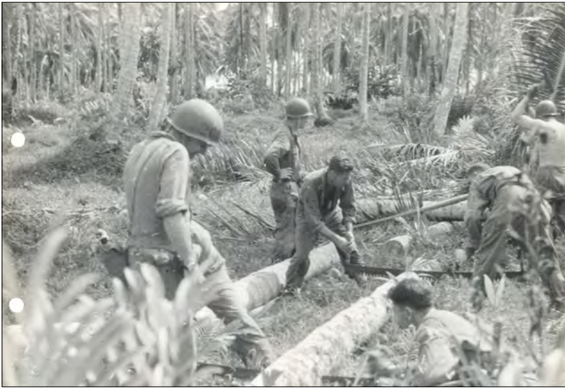
Rendova, July 1943. Showing 24th Construction Battalion men sawing coconut logs into proper lengths for corduroy log road construction. —From: Lest We Forget, Seabee Museum
