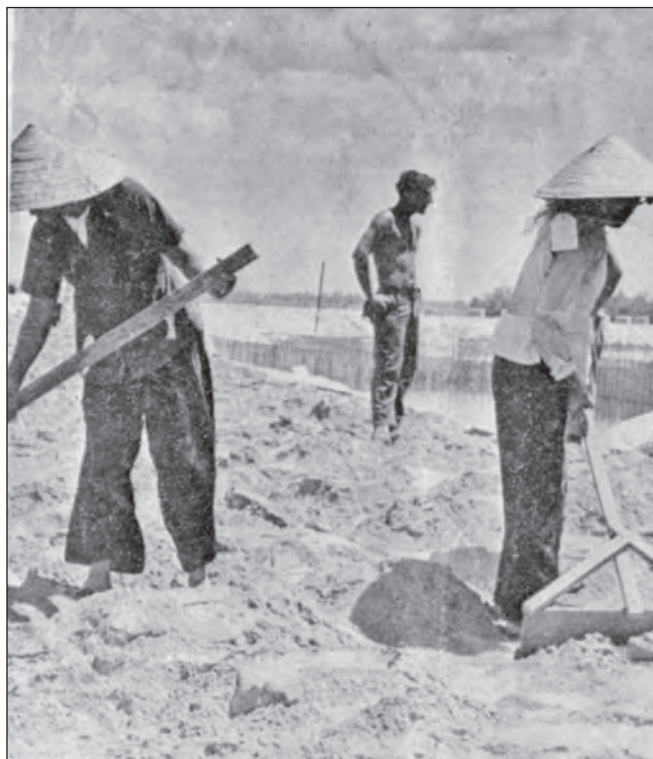
Dispatched trucks unload cement on Col Co Road and Vietnamese laborers spread the soil and cement. 40 such laborers are supplied to this job site. (Col Co Road job by MCB8 in 1968—or was it yesterday? kb) —Photo by R.F. COTTER
