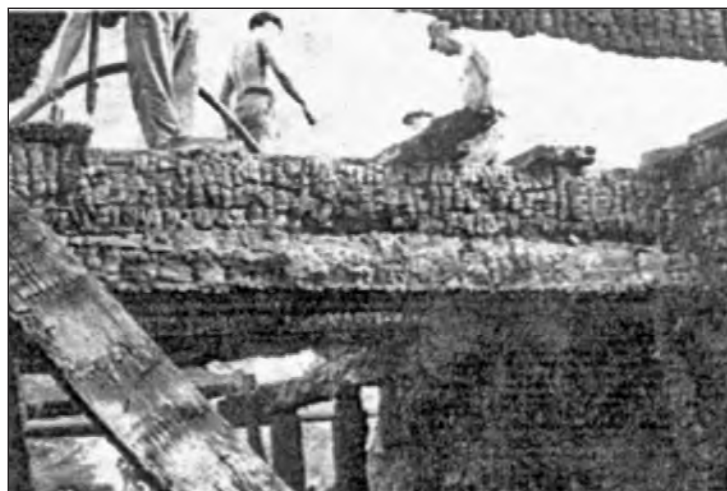
BUC Niemeyer and Crew moved to rebuild Bridge No. 6 on Col Co Road after being burnt by enemy fire. —Photo by B.A. Farley
