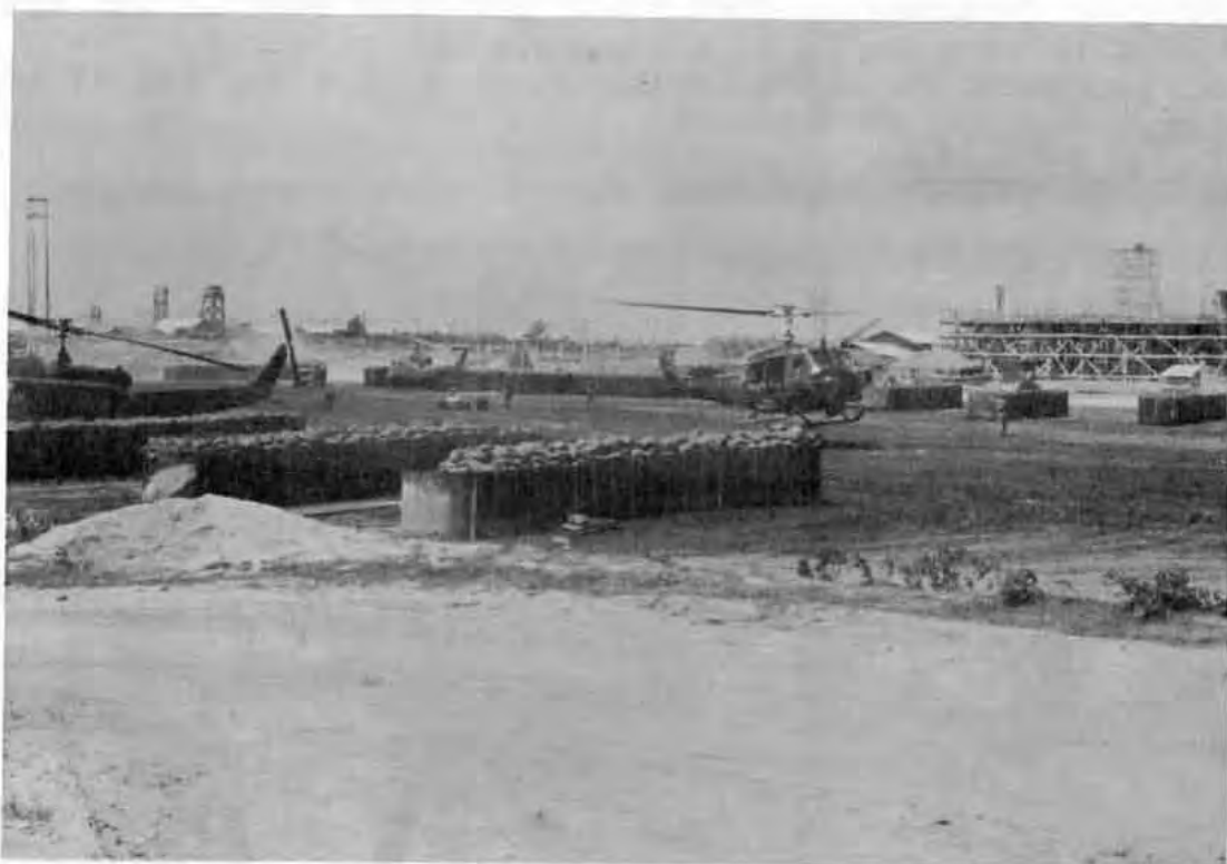
Helicopter landing zone constructed at An Hoa.
