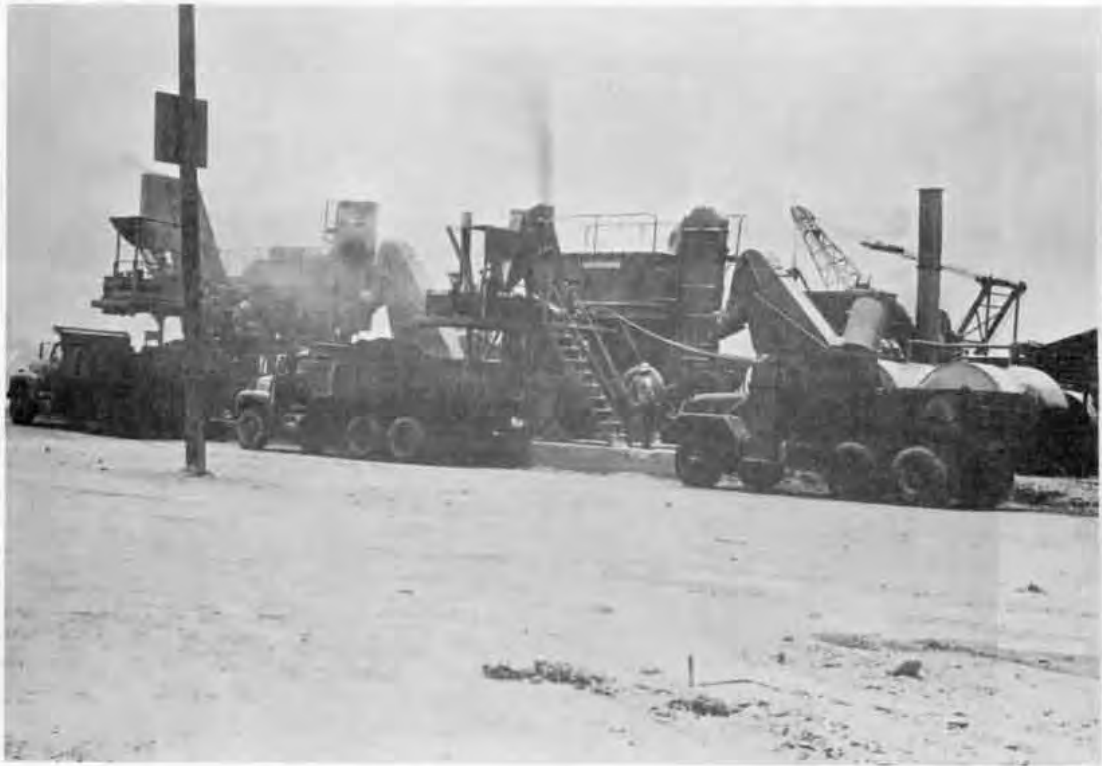
Detail Zulu asphalt plants in operation.
