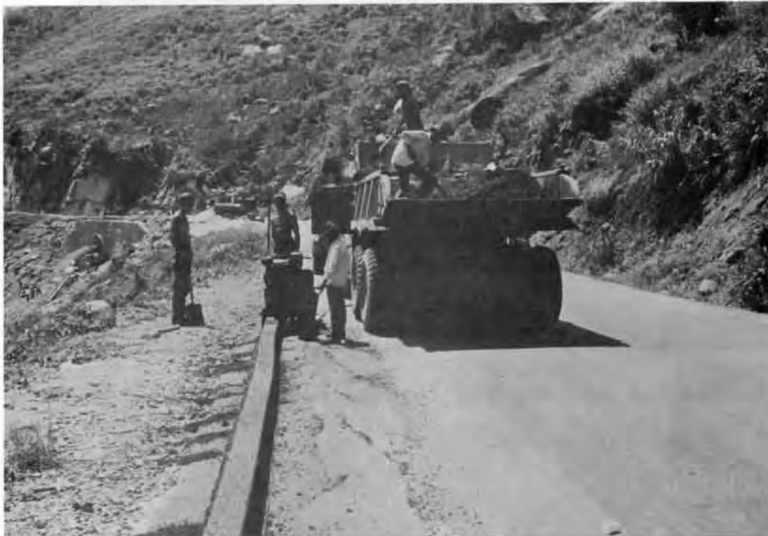
Placing Asphalt Curbing in Hai Van Pass for erosion control.
