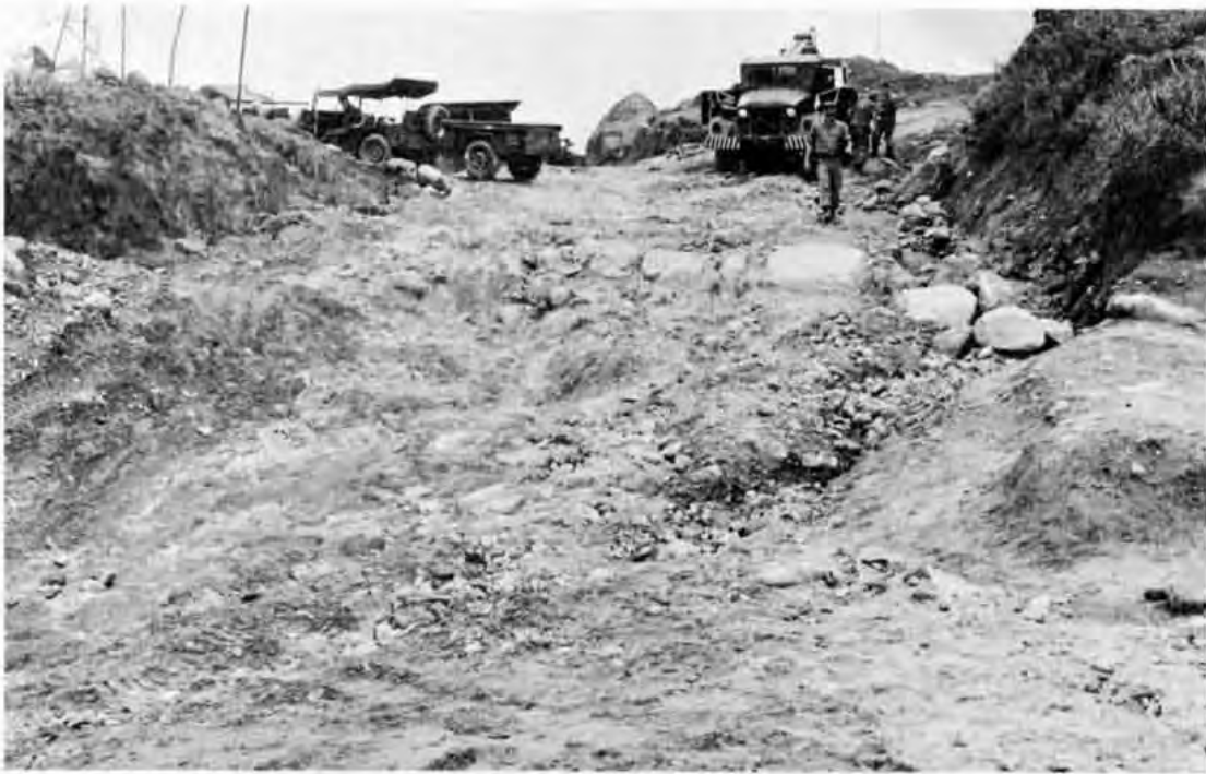
LAAM Battalion Road is cut through a hill to reduce the grade, this portion is typical of many areas of the road prior to reconstruction.
