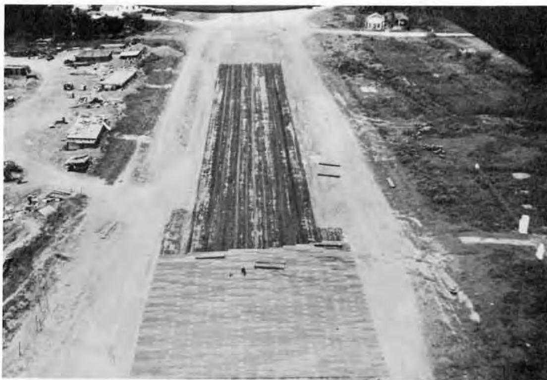
Tien Phouc airfield landing strip partially completed.
