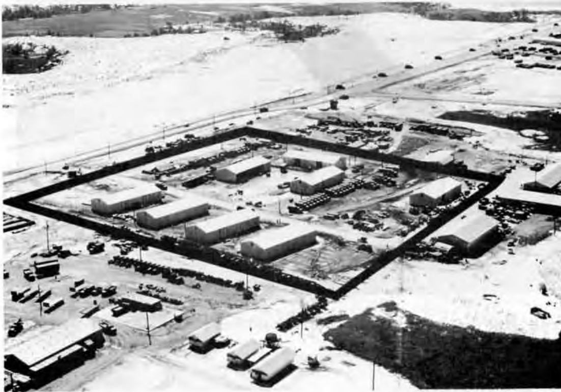
USMC Truck Company Cantonment constructed by NACB EIGHT.
