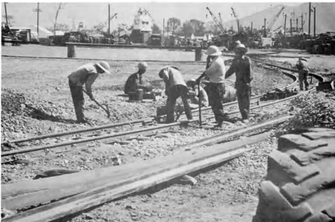
NMCB EIGHT provided surveying and equipment support for the railway installed by Vietnamese at the Bridge Cargo Storage area.
