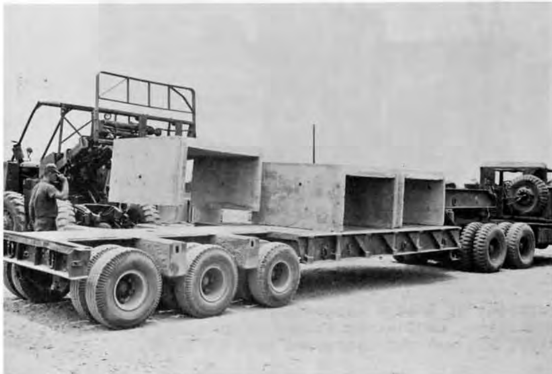
Precast concrete ditch sections to be installed at Bridge Cargo Storage area.
