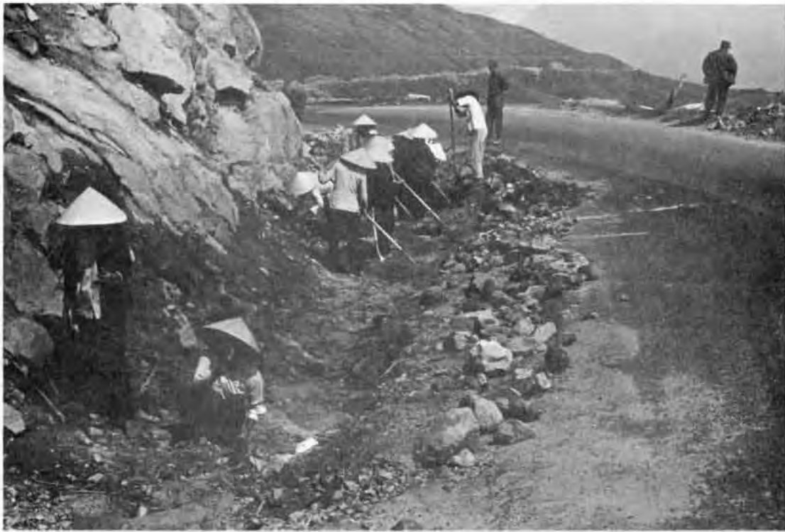
Vietnamese laborers preparing ditch for the placing of a concrete lining.
