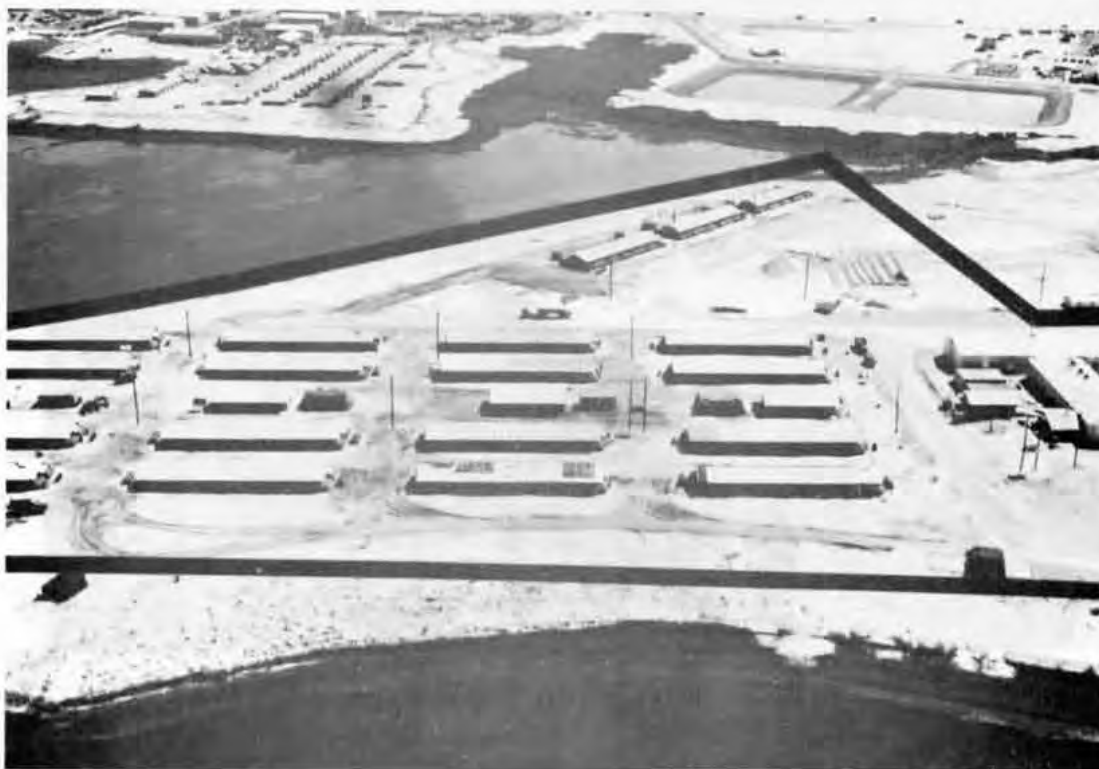
First FSR Vehicle Maintenance area, Camp Books. This work had been partially begun when taken over by EIGHT.
