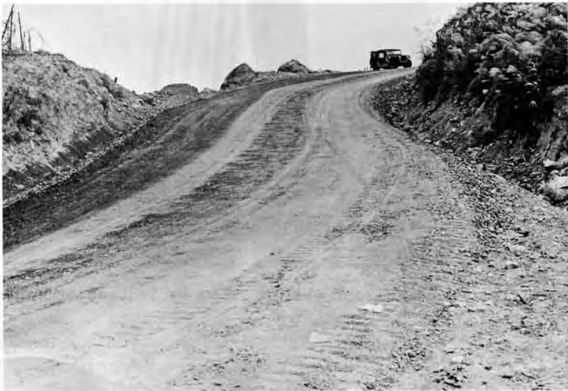
The cut areas shown in preceding photo after completion of roadway.
