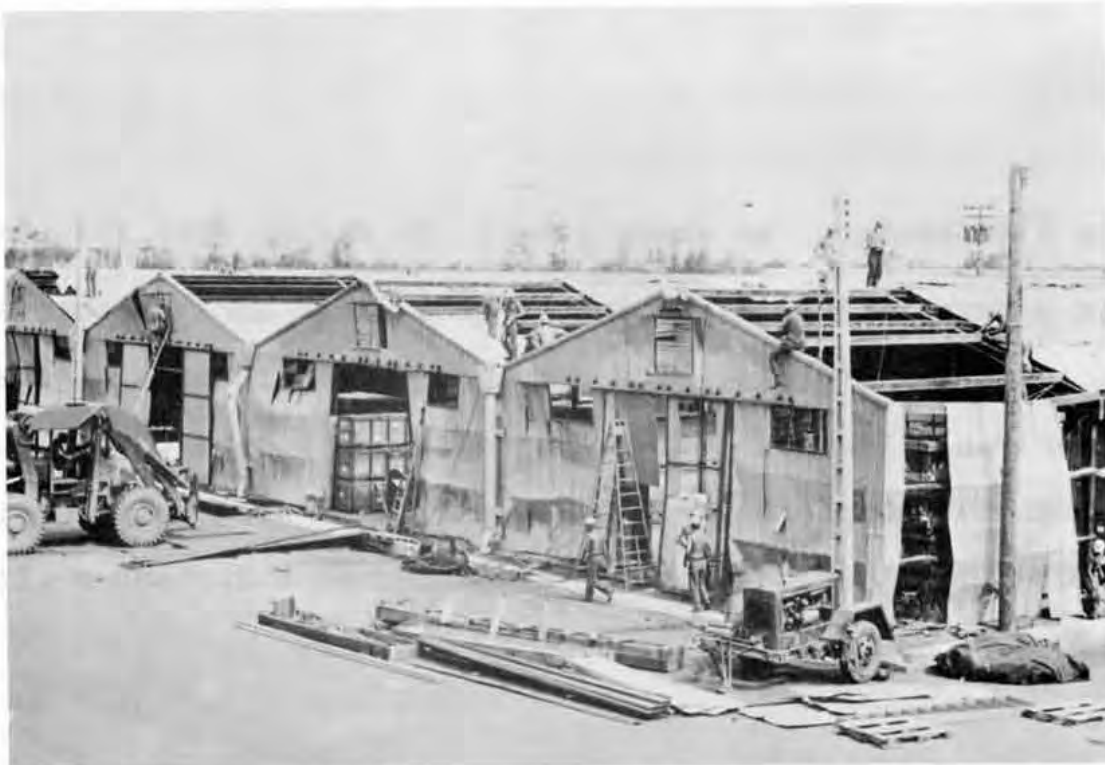
NSA Covered Storage during reconstruction.
