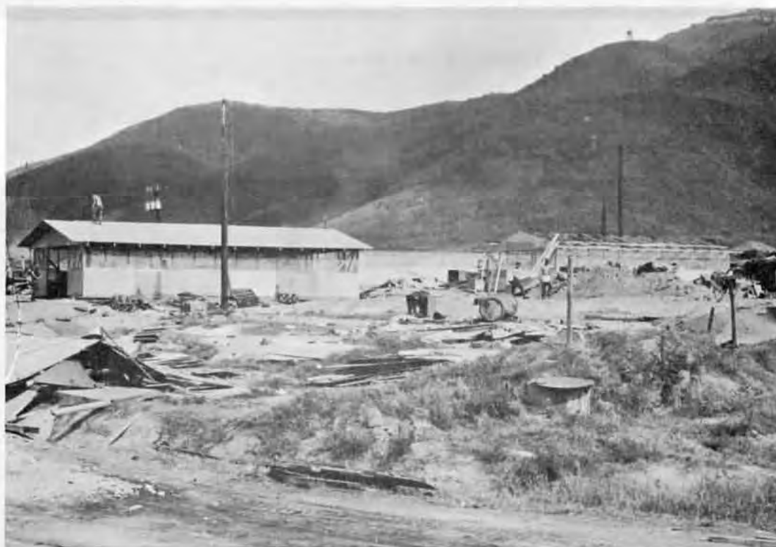
Reconstruction of 3rd MP cantonment in progress.
