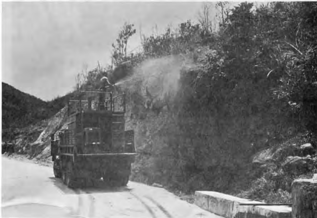
Applying Hydro Mulch in Hai Van Pass to control erosion.
