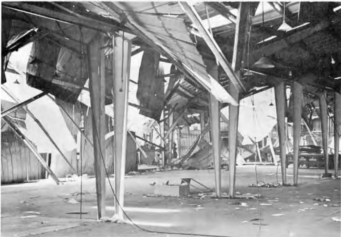
Freedom Hill Exchange Complex after blast from ASP #1.
