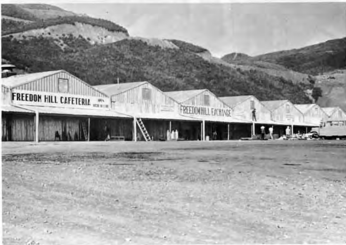
Freedom Hill Exchange after reconstruction by NMCB EIGHT.
