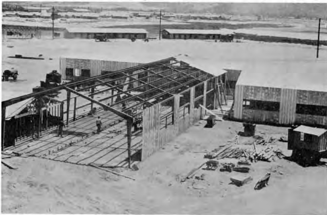
First FSR gallery under construction. BOQ's are nearing completion in the background.
