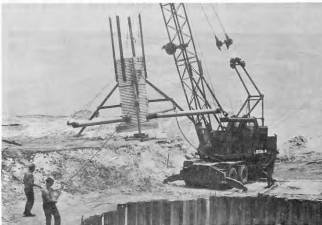
The water supply system infiltration gallery. Sheet piling cofferdam has been driven and sand excavated. The four-arm bottom section is being lowered into place, after which the sand pack was placed, top section installed and pile extracted, the hole filled and pump and piping installed.
