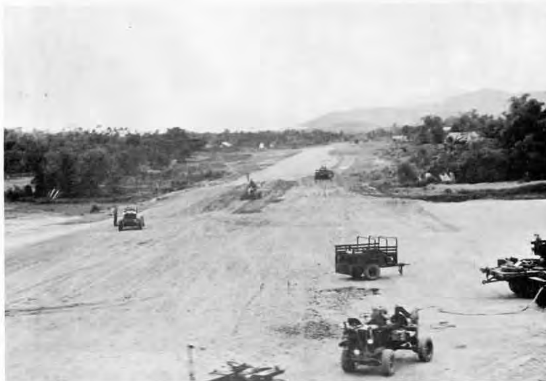
Airstrip grading at Tien Phouc airfield. Detail Victor up-graded the airstrip to compacted rock surface, then shot with asphalt.
