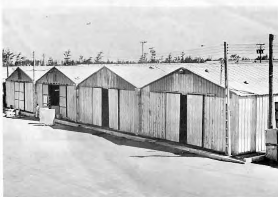
NSA Covered Storage warehouses after reconstruction.
