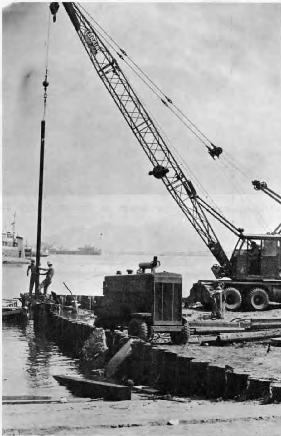
File driving at Bridge Cargo Ramp. This ramp was destroyed by ammunition explosions caused by an enemy rocket in February, and was reconstructed by NMCB EIGHT.
