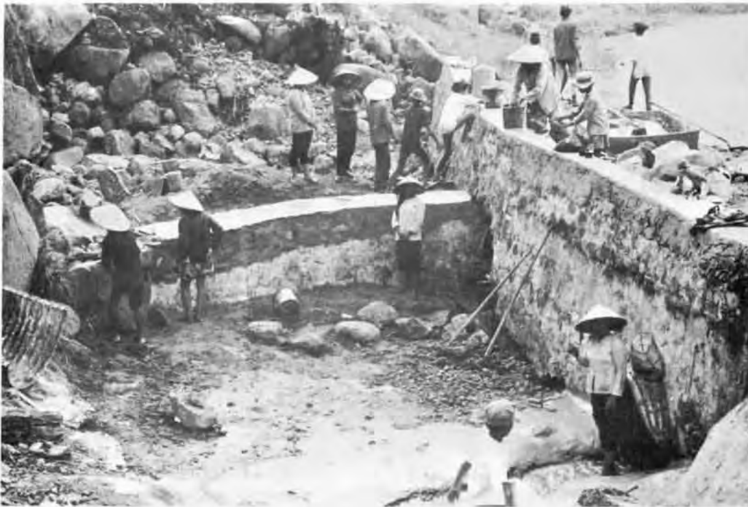
Vietnamese laborers working on drainage structure in Hai Van Pass.
