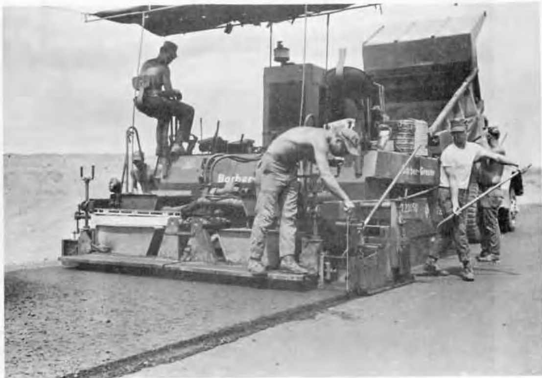
Paving of Highway QL #1
