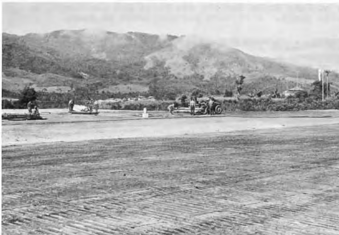
Men of Detail Sierra laying M8A1 matting of runway at Tien Phouc Airfield.
