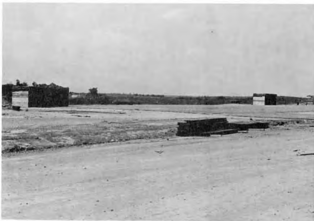
Bunkers and landing strip constructed by NMCB EIGHT at An Hoa.
