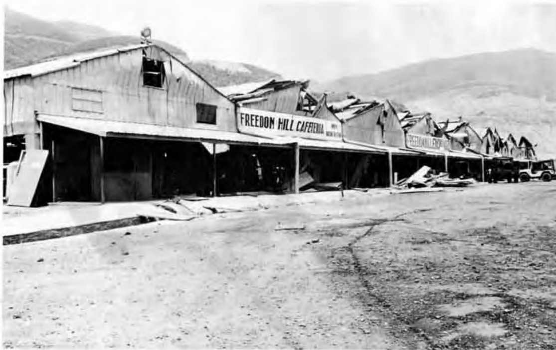
Extensive damage to Freedom Hill Exchange resulting from ASP #1 disaster.
