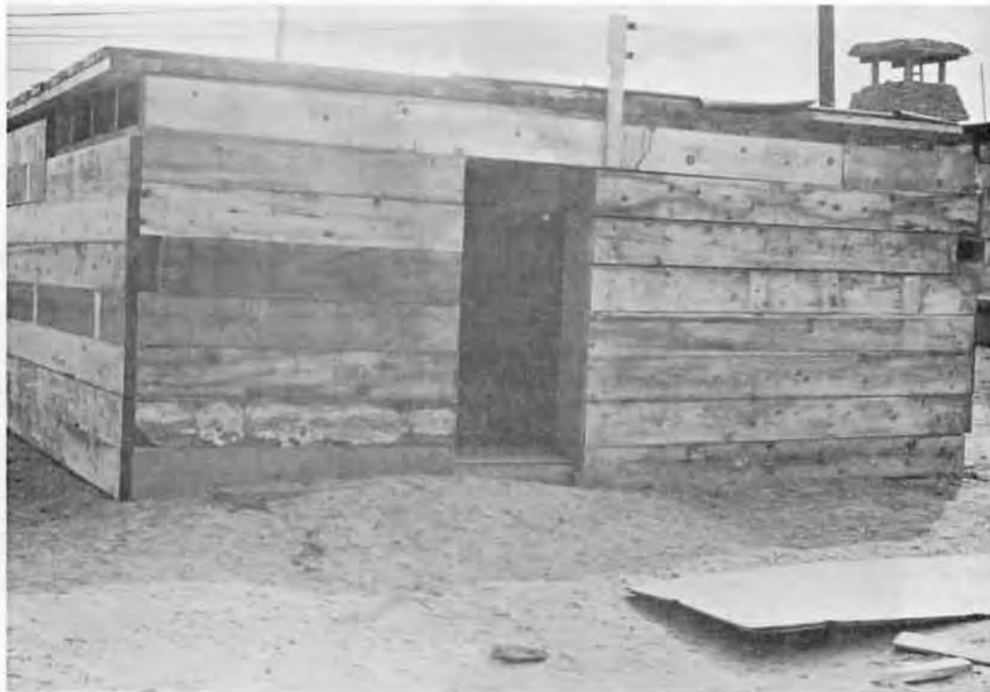
Typical bunker constructed for USMC at An Hoa
