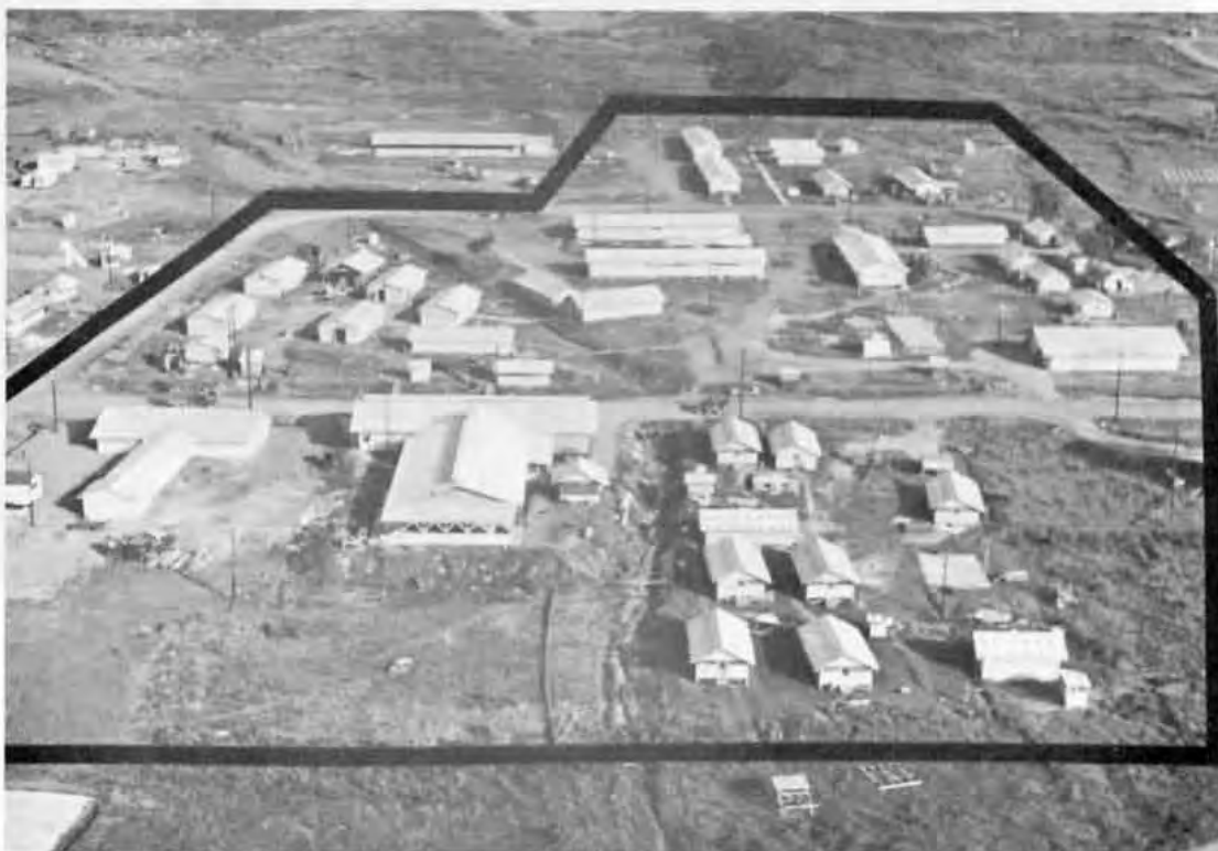
East side of 3rd MP cantonment reconstructed by NMGB EIGHT. Concession bldg., galley and living spaces are in the foreground.
