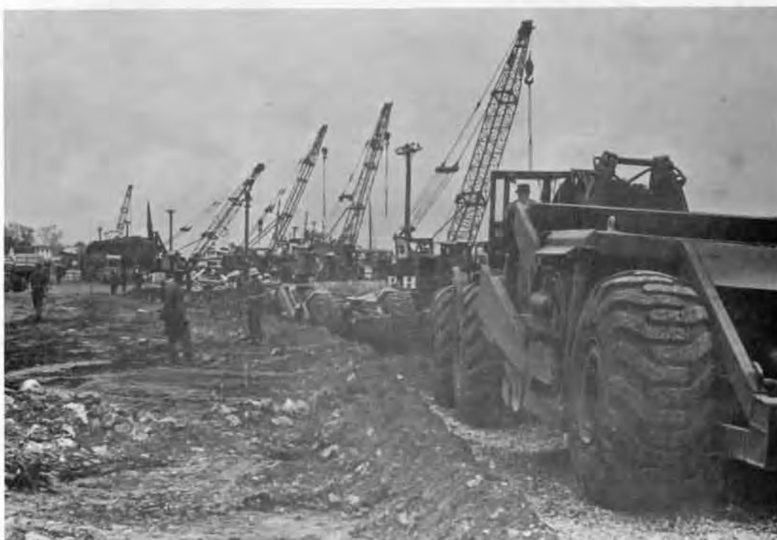
Placing crushed base rock in preparation for paving at Bridge Cargo Storage Area.
