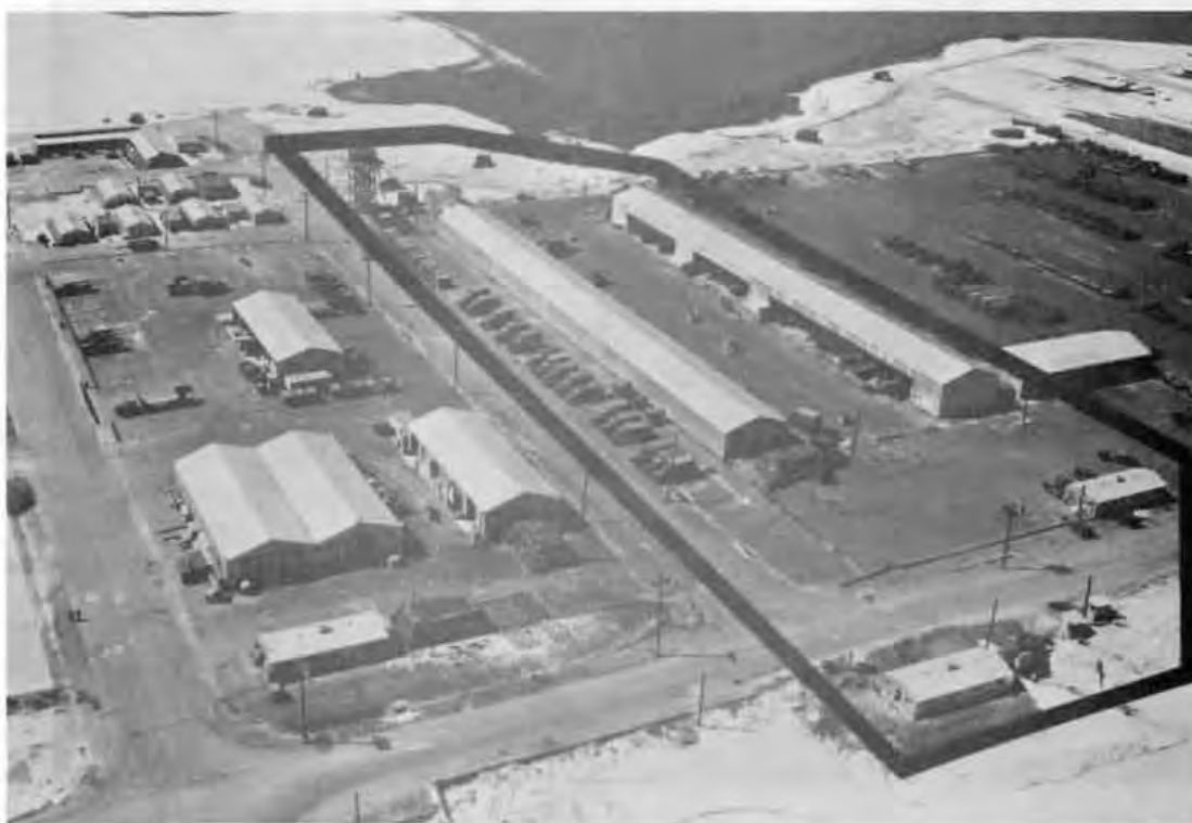
First FSR South cantonment with barracks, BOQ'S, head and shower facilities, and galley with water, sewage and electrical distribution systems.
