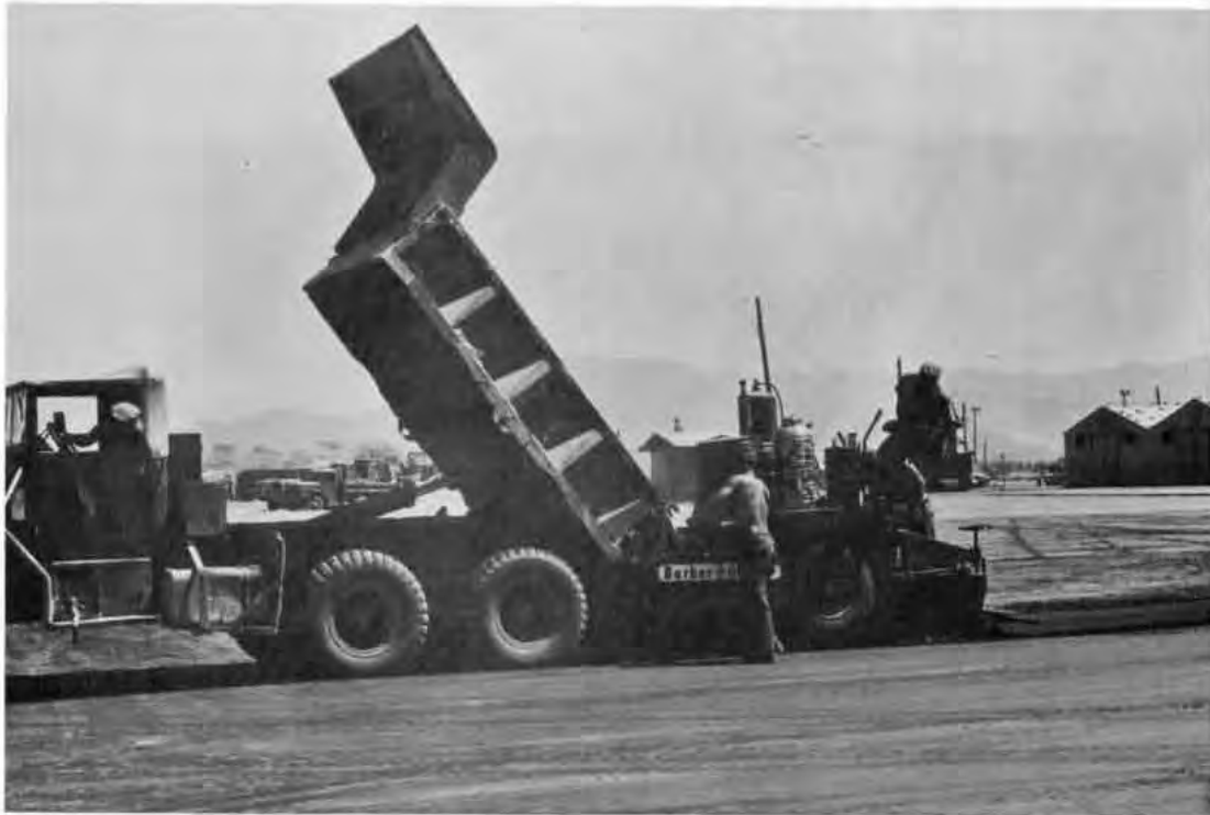
Asphalt paving operation in progress at Bridge Cargo Storage area.
