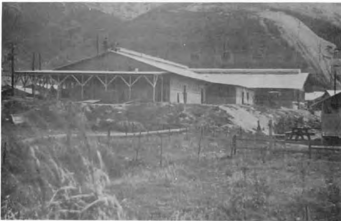
Third MP Galley reconstructed.
