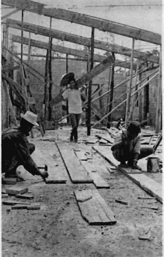
BEGINNINGS OF A VIETNAMESE CIVILIAN HOSPITAL — Forms go into place (above) for concrete beams used to support the hospital's roof. Vietnamese workers put the concrete forms together (below). —Photo by PH3 R. F. Cotter
