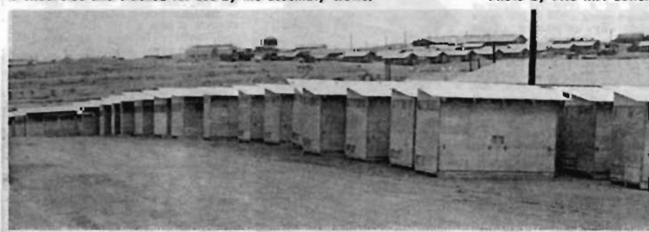
ALL PRE-CUTTING is done in Camp Wilkinson's pre-cut yard for the construction of showers and latrines for the Army. Production lines swallow the camp as Battalion personnel work 'round the clock for maximum output. —Photo by PH3 R. F. Cotter
