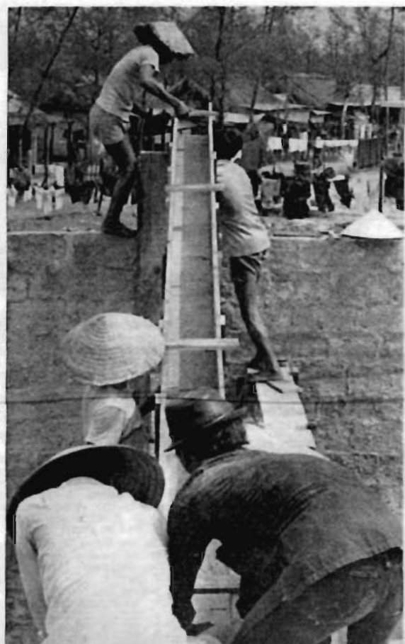
THE HOSPITAL DESIGN required several structural techniques previously unique to the Vietnamese builders, shown here placing formwork for roof beams. Photo by PH3 R.F. Cotter
