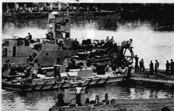
BULLDOZER AND TUGBOATS were used to get the YFU across the causeway and into deeper waters after being swept over by typhoon winds.
