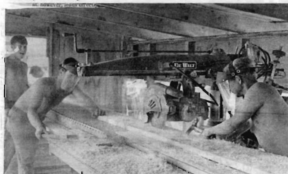
CHARLEY COMPANY'S PRE-CUT YARD was kept in operation 24 hours per day. The lumber was cut to exact size and stacked for use by the assembly crews. Photo by PH3 R.F. Cotter
