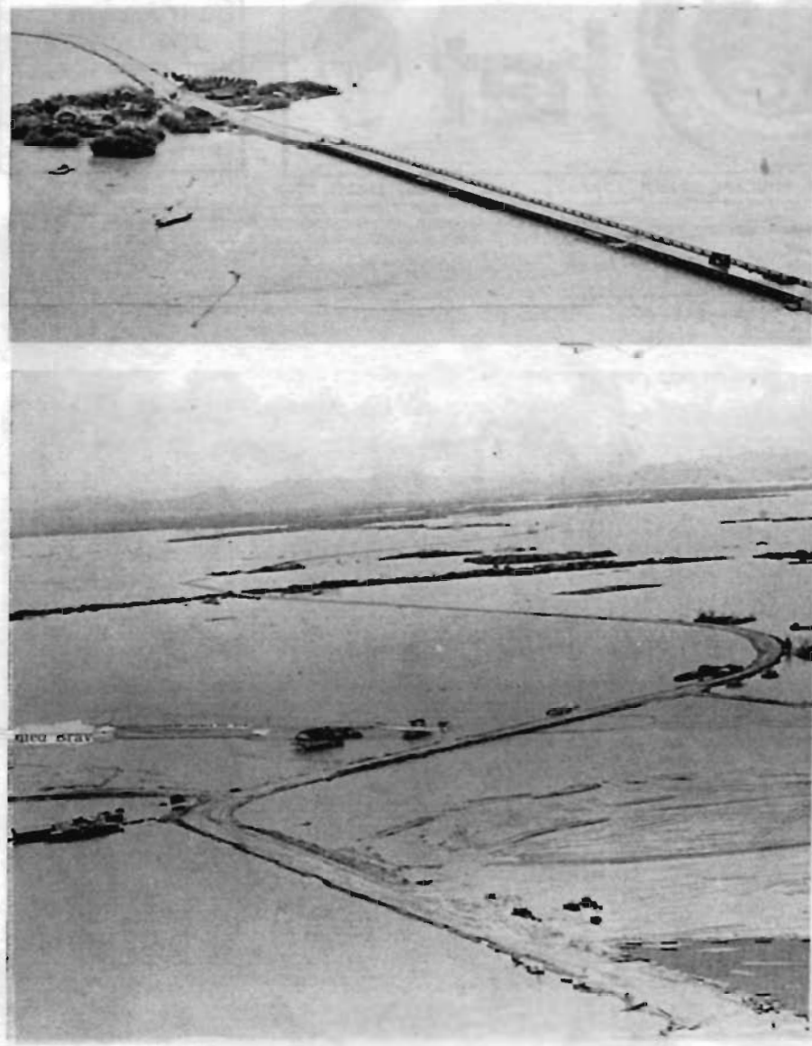
Bridge No. 10 on Col Co Road (top), normally 8 to 8½ feet above water level, resembles a floating pontoon crossing during the Hue flood of Sept. 5 and 6. Col Co Road (bottom) snakes its way across water-filled rice paddies. The flood reached heights of over 11 feet above normal in some areas.
