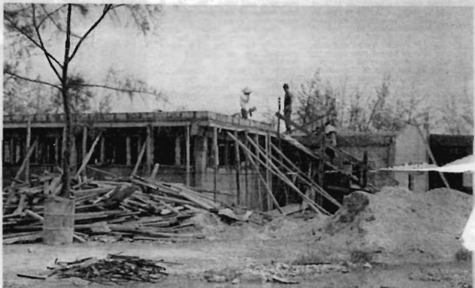
EA2 R. STEVENS VISITS THE HOSPITAL SITE. Makeshift formwork and braces were made utilizing all sizes and shapes of available lumber. Photo by PH3 R.F. Cotter
