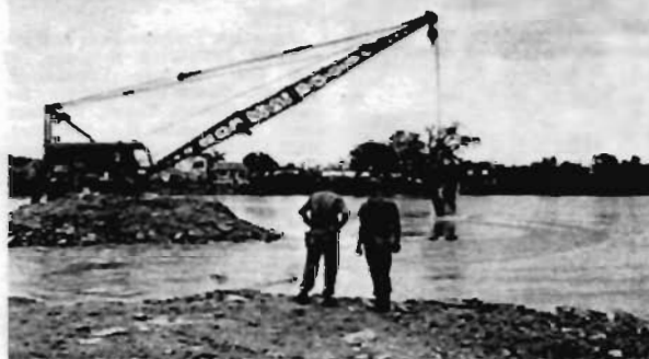
CLAM BUCKET removes rock and broken concrete from hole carved in Col Co Road causeway by stranded YFU.
