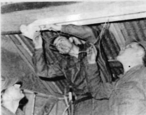
BRIGHTNESS BY BRAVO (By the way, thanks!) — CEW2 W.R. Hallam, CN W.J. Gentry and CES2 J.W. Williams install fluorescent light fixtures in the battalion's Public Affairs Office. The men of Bravo Company take care of almost all camp maintenance plus project utility work.
