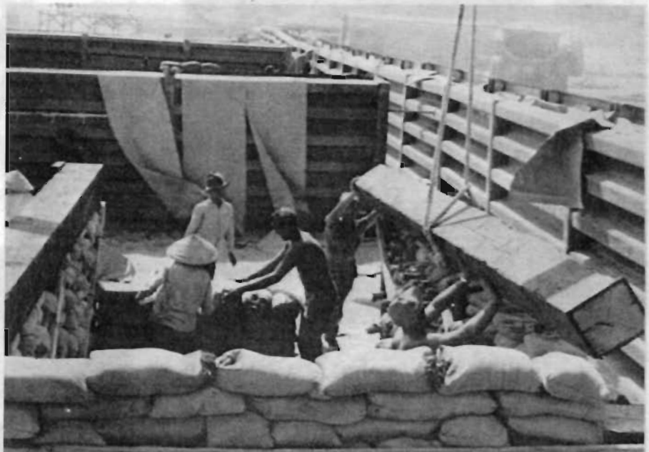
DELTA CO. MEN ON PACV SITE—Vietnamese laborers and SEABEE builders D.J. Josephson, T.H. Zopfi and J.O. Kelly work together to build bunkers and revetments at the high priority PACV project site completed June 29.
