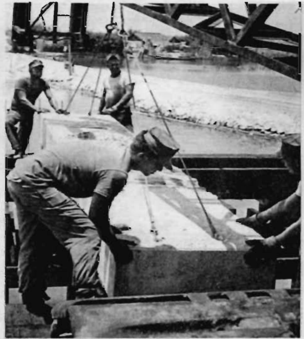
PRE-FABRICATED IN DA NANG, RVN—Concrete fire breaks are placed into position on Bridge 10 in early July by Bridge Crew members BU2 D.S. Ewald, CN D.L. Smock, (foreground) BUCN R.E. Bailey and BU2 H.W. Throppe. Breaks weigh 7,000 lbs each.
