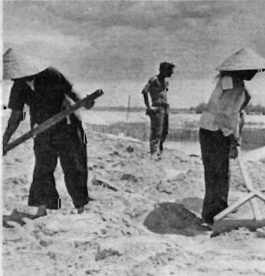
Dispatched trucks unload cement on Col Co Road and Vietnamese laborers spread the soil and cement. 40 such laborers are supplied to this job site.
