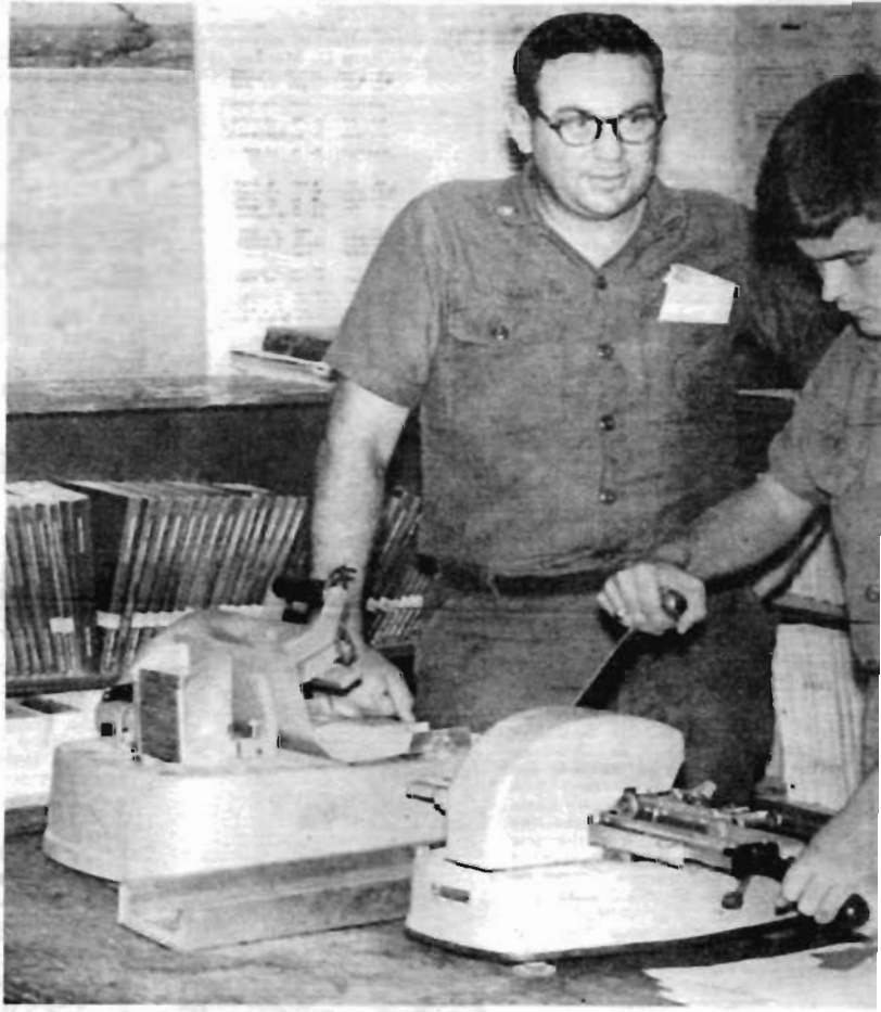
THE EMBOSSE is used to print the name, rate, serial number, active duty base date, or branch of service of each man. CEC Russell verifies information embossed on each plate. The printer affords speed in preparing any list, whether original, carbon or stencil.
