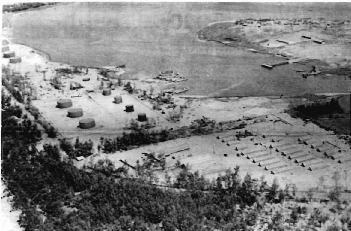
NAVAL SUPPORT ACTIVITY CANTONMENT consisting of living quarters, 500-man mess hall and galley, Post Exchange, fire house, laundry, dispensary and fuel farm was constructed by MCB EIGHT personnel in three phases. The three phases included building of huts and utilities and soil cementing. The complex features a 16-point well system which draws water for a 500-barrel steel tank resting on a 36-foot timber tower.
