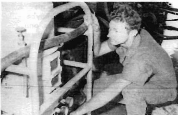
ON THE JOB FOR BRAVO COMPANY—UT3 L. D. Wyatt Jr. turns the valve back—flushing the filter for the water purification process in Camp Wilkinson.
