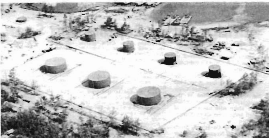
FROM COL CO ISLAND BY THE SEA—The Tan My fuel tanks feed the pipeline which carries the fuel to a pumping station near Hue where the fuel is routed north and south.
