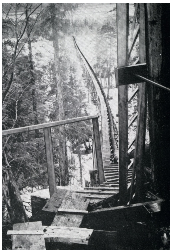
Flume box and pipe line built at Sitka Alaska to provide fresh water for the Naval Air Station. This work was done by the 22nd NCB. (Official U. S. Navy Photo)
