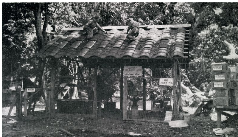
There is nothing Seabee's can't do with an empty gasoline drum. Here the empty drums are being converted into a roof for a jungle machine shop. (Official U.S. Navy Photo)
