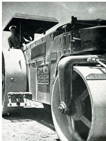
Like any other great highway, the roads to Tokyo are built with heavy equipment. Here is a 40-ton roller on an airstrip in the Solomons. (Official U.S. Navy Photo)
