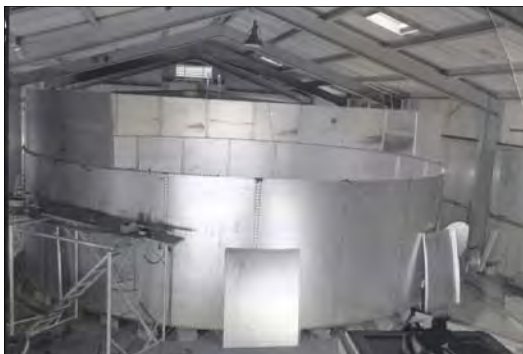
55,000 gallon water tank and interior view of the salt water distillation plant.
