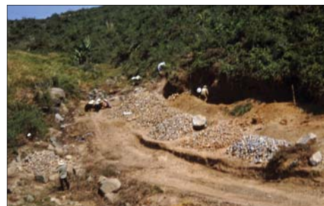
MCB-8 allowed the locals to break rock (rip/rap), by hand, and sell them to the battalion for road construction
