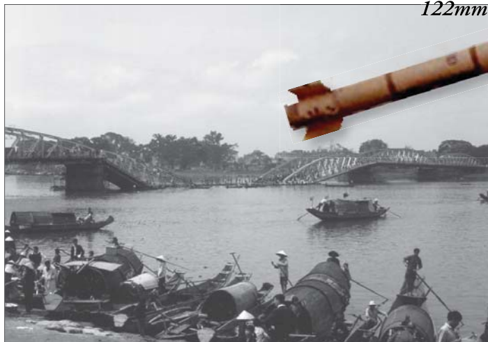
Railroad Bridge over Perfume River blown up by NVA during TET. (Battle of Hue was raging). MCB-8 made emergency temporary repairs by bridging a connection between the downed trestle sections.
