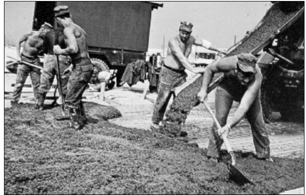
Men of Charlie Company pouring concrete during the 1969 deployment in Danang
