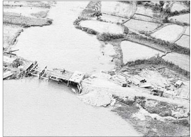
60 Ton Timber Bridge Project near the Vietnamese village of Bien Son constructed during the Chu Lai deployment
