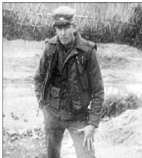
BM3 Ray Longaker Jr. at the MCB-8 60 Ton Timber Bridge Project at Bien Son.
