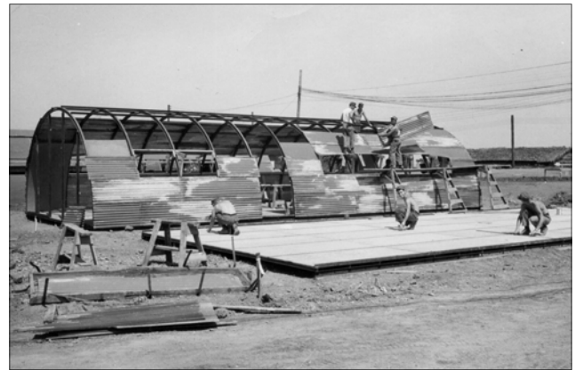
Charlie Company constructing a Quonset hut in Chu Lai 1967.
