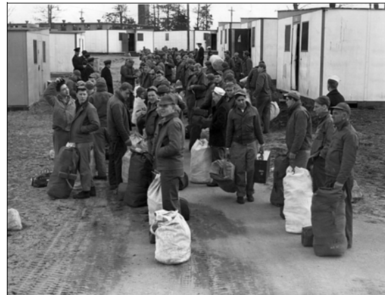
Dick's "D" Company leaving for NAS Bermuda to build seaplane ramps. "After this deployment I got back home and took my new wife to Niagara Falls and Grand Canyon on a honeymoon." 2/28/53
