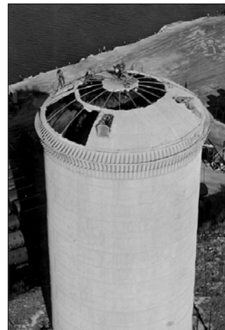
A group of EIGHT Steelworkers actually volunteered to take out this old reinforced concrete silo on a quay in the Bay at Gitmo. It was considered a flight hazard. Other Battalions refused. These guys tied themselves on and jack hammered the concrete out that they were standing on 80' or so above the ground and then burned the steel rebar off. 1952
