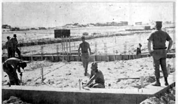
THE OVERSEER—BU1 S. Rosenswig, (R), looks over the hangar project, which his crew is working on for MAG-12. The only question is, "Do they have a complete hangar?"
