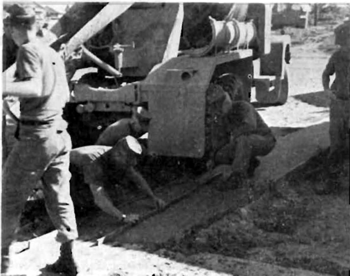
"YES SIR, I THINK THIS IS THE WAY—(L-R) YN3 John Miller, BU1 W.C. Legat, ENS P. E. Loberg, and EAD3 F. H. Johnson do a little base maintenance on a sidewalk by their Ops Office. A TM was called in to pour the three feet of cement.
