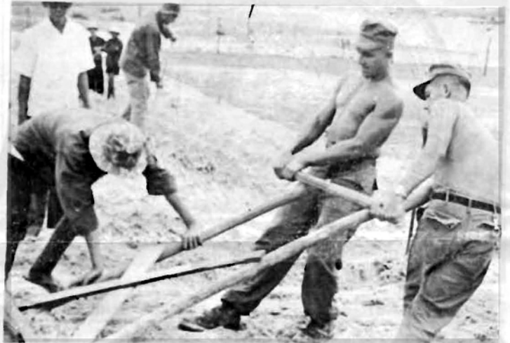
BUR2 J. R. Maynard (L) and BUL2 F.J. Klein with the help of a few Vietnamese use a tool designed to level the sand in preparation of the foundation of a school. USN MCB EIGHT played a vital roll in the construction of the school in Chu Lai.
