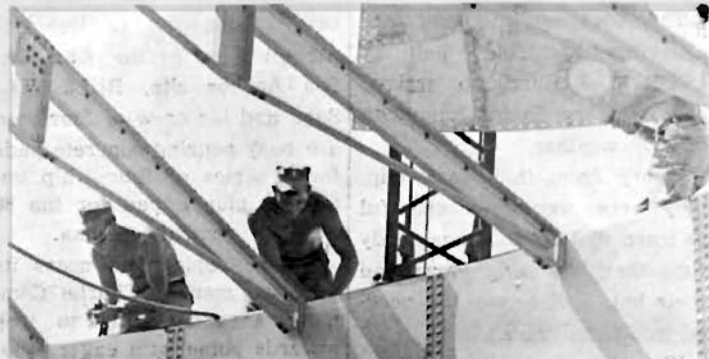
"THIS REMINDS ME OF MY ERECTOR SET" — The first metal sheet for the roof of one of the POL tanks is brought in as Seabees of Charlie Company make the final preparations for its installation.
