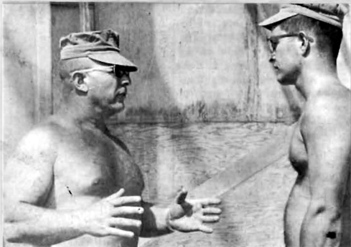
"I DON'T KNOW HOW TO TELL YOU THIS, BUT WE HAVE TO BUILD THE WHOLE HANGAR ONE FOOT LONGER."—BU1 S. Rosensweig and BUL2 L.A. Carigan discuss a minor construction problem on the MAG-12 Hangar project.
