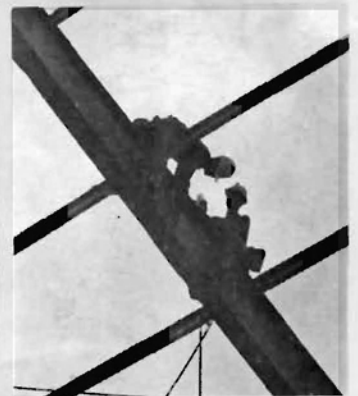
WORKING INTO THE TWILIGHT HOURS are two construction men from Charlie Company as they add the finishing touches to the frame of the MAG-12 hangar.
