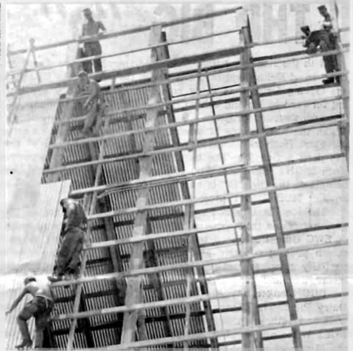
"GONNA BUILD A MOUNTAIN" — Construction men of Charlie Company tin the roof of the NSAD Chapel which will rise 41 ft. in the air when completed. The A-frame structure will be able to accommodate over 200 people.
