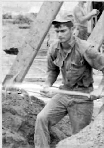
"THEN HE HANDED ME THIS PICK, AND THE NEXT THING I KNEW . . .!" — UTW2 D.R. Epplert digging a ditch prior to the installation of the drainage system of the NSAD Chapel. Bravo Company installed the electrical and plumbing facilities for the structure.
