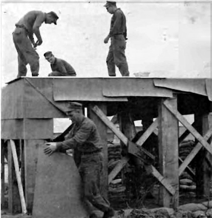
THE OVERHEAD of the "H" Co. Command Post nears completion, as YNC M. S. Kofoed, (on ground) R. F. Corn, EAS3, (L), BUL2 J. O. Frye, (C), and G. W. Grimshaw EASCN (R), put down the insulating paper and tin, which will be followed by sandbags. (Photo by JO3 J. C. Davis)
