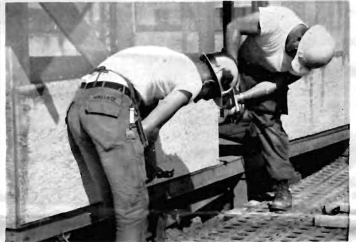
CN R.A. WALLACE and BUL3 J.J. Defeo, Jr., Delta Company, work on one of the many strongback huts that were re-tinned by EIGHT, at the Seventh Marine Motor Transport Battalion. (Photo by PH1 C.V. Wade)
