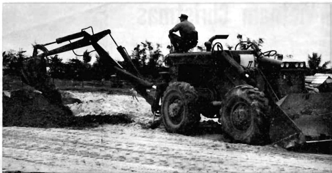
A HELPING HAND —EON2 W. N. Epperson, of USN MCB EIGHT Alpha Company, digs the helpful drainage ditch, that serves two purposes. The first purpose is to drain flooding waters from one of MCB EIGHT's projects in Tam Ky, Vietnam, and secondly to keep a rice paddy flooded for the local Vietnamese. (Official Photo by PH2 B. J. Gaetano)
