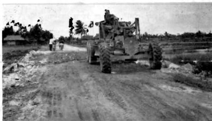
EON2 R.M. DEMPSEY , Alpha Company, operates a grader in the road repairing operations on Route One. (Photo by PH2 B.J. Gaetano)
