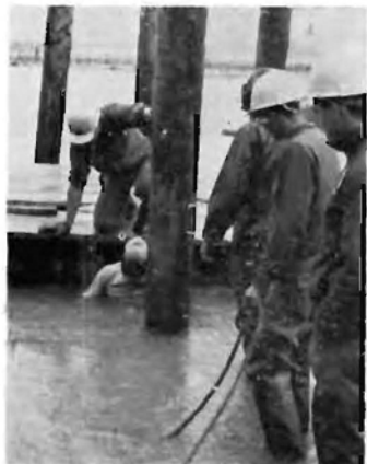
BATTALION DIVER BUR2 J.R. Schauffhauser, Jr., prepares to make his descent, to help set the piles at the timber bridge project on Route One.
