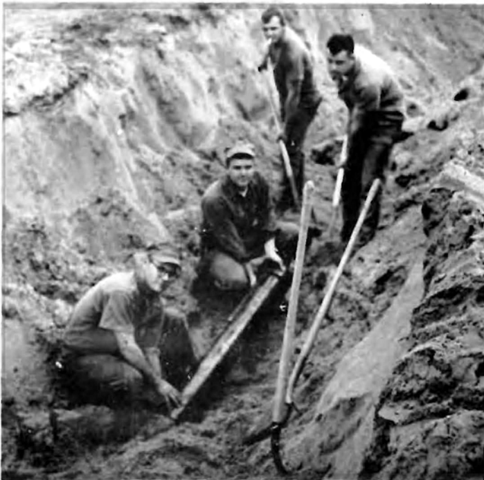
NO HELP NEEDED—(front to rear) CN R.A. Holbrook, UTA3 K.W. Richards, UTACN C.R. Schropp, and UTP3 J.P. Sullivan, Jr. put in a septic tank pipe line at the Naval Support Detachment. (Photo by PH1 C.V. Wade)
