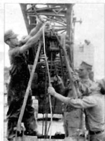
THE JOB IS ALMOST OVER —(L-R) EON3 Al Price, EO1 R. N. Rader, and CA E. R. McBroom, rig a clam shell bucket at the bridge One, as their job comes to an end.
