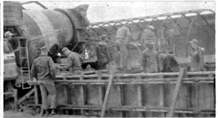
A BIG 'D' crew prepares to make another concrete pour for another quonset hut at the First Force Hospital.
