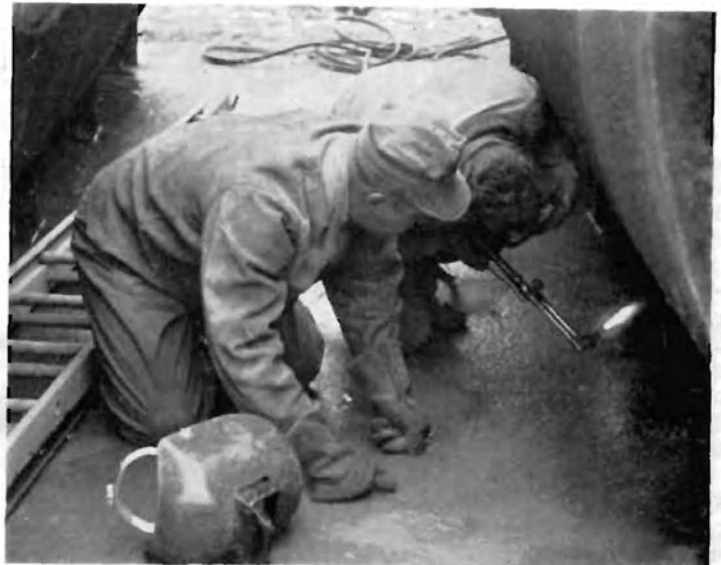
SWFCN Ron Skalka, (L) and SWF3 C.M. Harrington, do the welding on the four underground 5,000 gas tanks, which "C" Co. is installing for the NSD gas station.
