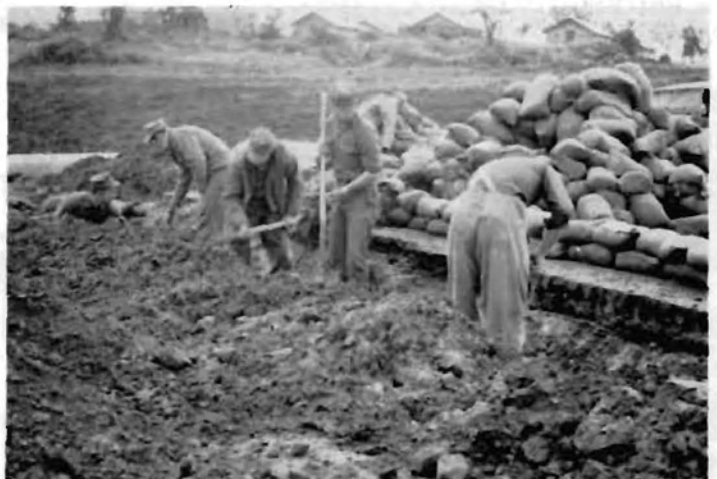
EVERYONE DIG — A "C" Co. crew, under BUR2 C. V. Brooks (second from Left), works on a drop inlet at MAG-36, for water drainage. (L-R) CN W.H. Smith, Brooks, CEW2 W. L. Whitaker, BUL3 P. C. Planky, and BUL3 W. L. Sack.
