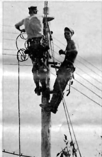
POWER TO SAVE LIVES—CEP2 J.C. Volk and CEP2 C.E. Hopkins installing one of the key links in the electrical system that will power 1st Force Hospital.
