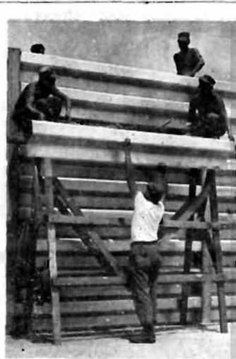
THE LAST PIECE OF SIDING is placed on one of the revetments signaling the end of an extensive and record breaking project at MAG-12 accomplished by the men of Delta Company. Shown here are: (clockwise from 10) BUR2 J.E. Womack, CEW2 J.T. Wasson, CEW2 E. R. Sterbinsky and CEW2 J.M. O'Connell.
