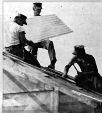
HUT ADDITION —BUL2 L.W. Rupp, BULCN L.W. Steele and BUL3 R.G. Luce begin installing corrugated tin roofing on one of the hut additions in EIGHT's camp. . .
