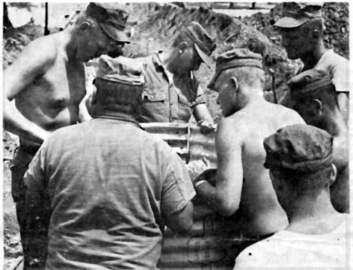
I DON'T KNOW WHAT IT IS, BUT AT LEAST WE'VE GOT IT TRAPPED—(L-R) UTACN W.A. Sahl, UT1 A.E. Alcalá, UT1 J.A. Young, UTP3 T.R. Reynolds, UTWCA V.L. Peterson, UTACN F.C. Garcia, Jr., and EON3 D.D. Emerson, Jr. prepare to install a manhole at 1st Force Hospital.
