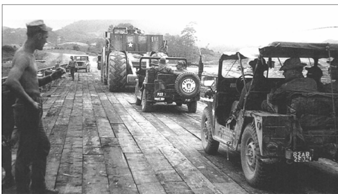
The men of EIGHT completed major repairs to a pontoon bridge spanning the Perfume River thus maintaining access to the SEABEE rock crusher at Nam Hoa.
