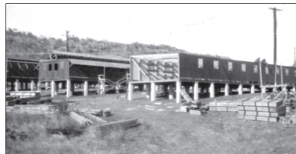
The Builders at work on their future homestead—Feb. 1952.
