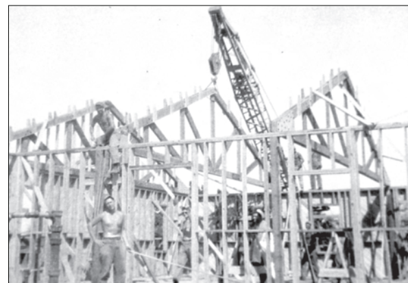
Setting the trusses. I helped slap the trusses together.
